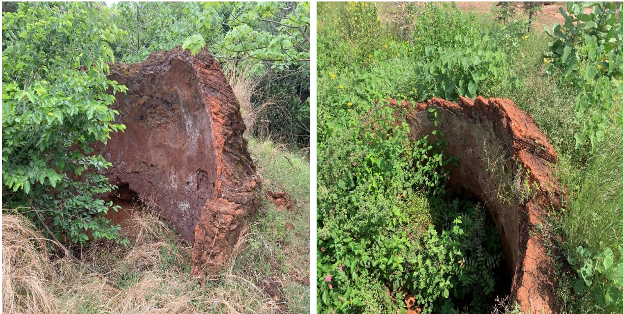
A dilapidated furnace at a glass bangle manufacturing site in Pavagada Taluk, as previously discussed in the Channapatna chapter.
