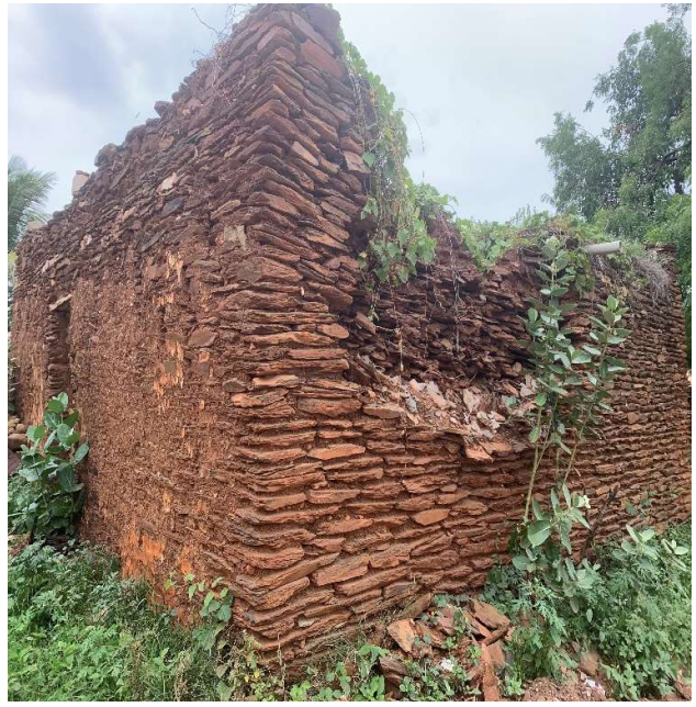
An old dilapidated house with walls built using talcose argillite slate for masonry work.
