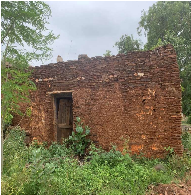
An old dilapidated house with walls built using talcose argillite slate for masonry work.
