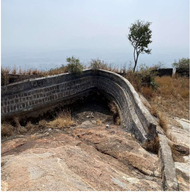
Clockwise from top left: 1 - View of Garudanagiri village from the top of the hill; 2 - Defensive fort wall ramparts atop the hill; 3 - The final fort wall gate at the summit; 4 - A 'done' masonry structure built across the ridges to collect rainwater, serving as a waterbody for use in olden days.
