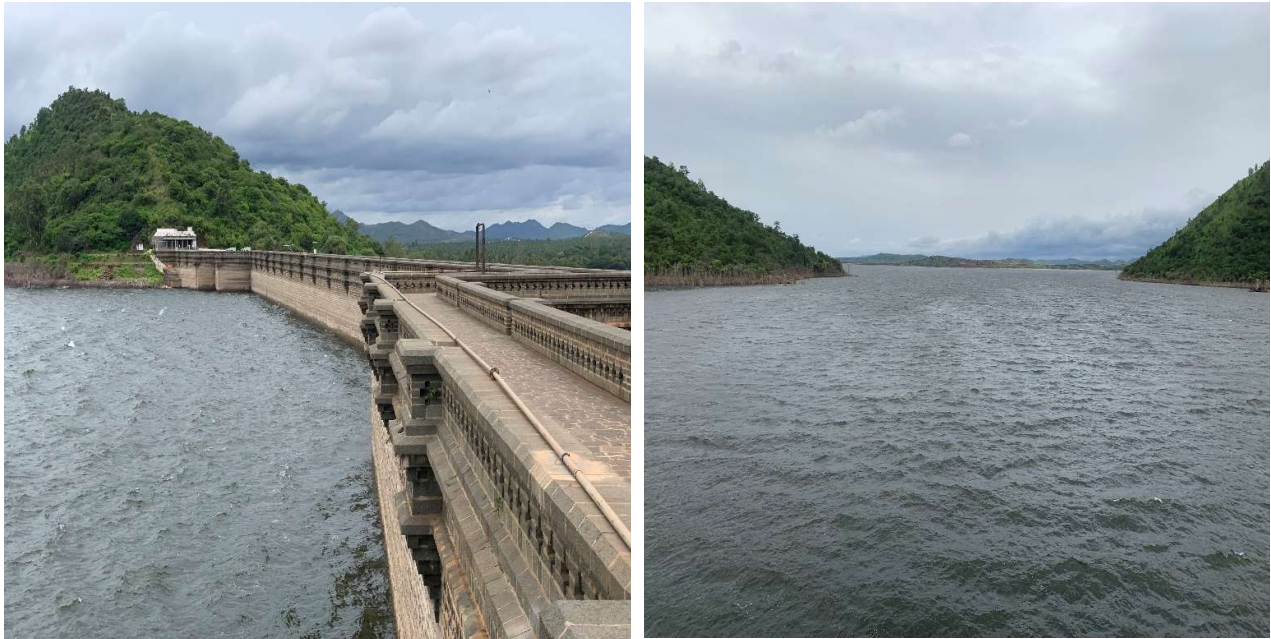
Clockwise from top left: 1 - Masonry work of the dam from the base; 2 - A marble tablet with information on the project, initiated in August 1898 and completed in August 1907 in the Marikanive Valley, led by Regent Queen Maharani Kempa Nanjammani Vani Vilasa Sannidhana; 3 & 4 - Views of the Vanivilasa Sagara Dam.
