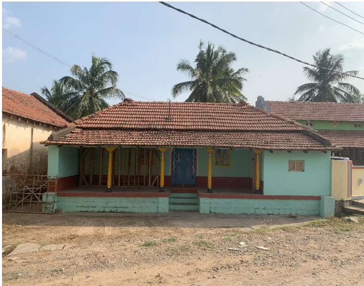
A Traditional Mysore-style Village House with a Clay Tile Roof and Wooden Pillars Supporting the Veranda Porch. The semi-circular shaped clay tiles, once common, were later replaced by Mangalore tiles with modernization.
