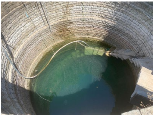
A traditional well with outer walls built using locally available granite stones is now equipped with an electric pump for water extraction
