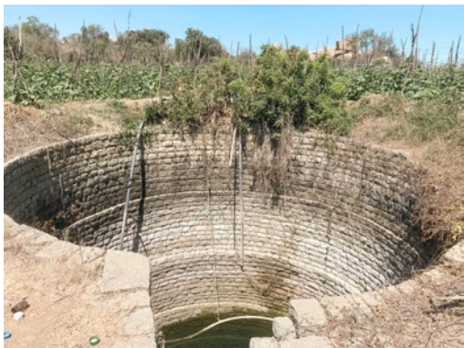
A traditional well with outer walls built using locally available granite stones is now equipped with an electric pump for water extraction
