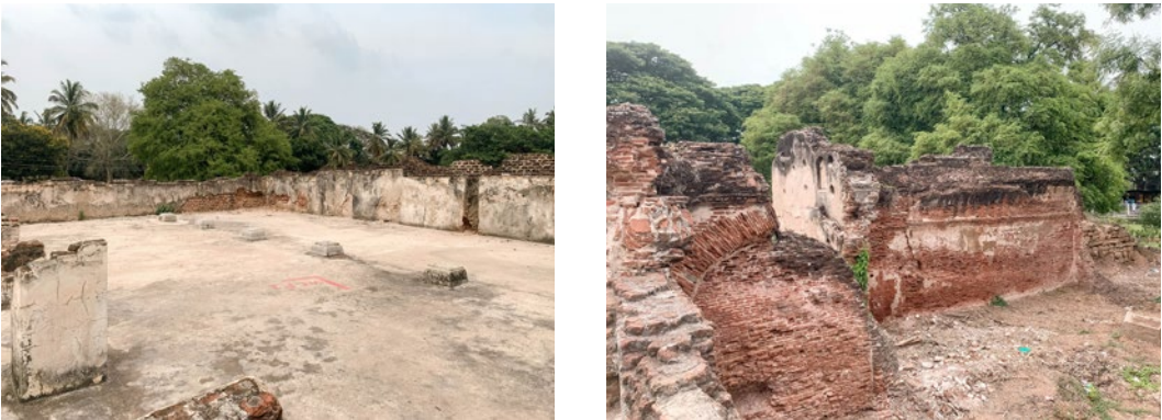
Views showcasing remnants of the once grand structure, including fragmented walls and foundations that hint at the palace’s former splendour before its dismantling between 1807-1809 AD
