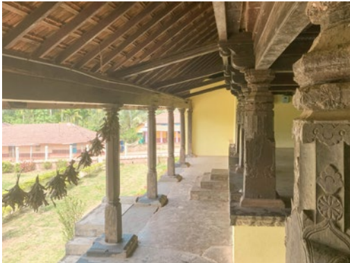
Keladi period architecture featuring wooden log pillars at the courtyard entrance paired with modern roof tiles
