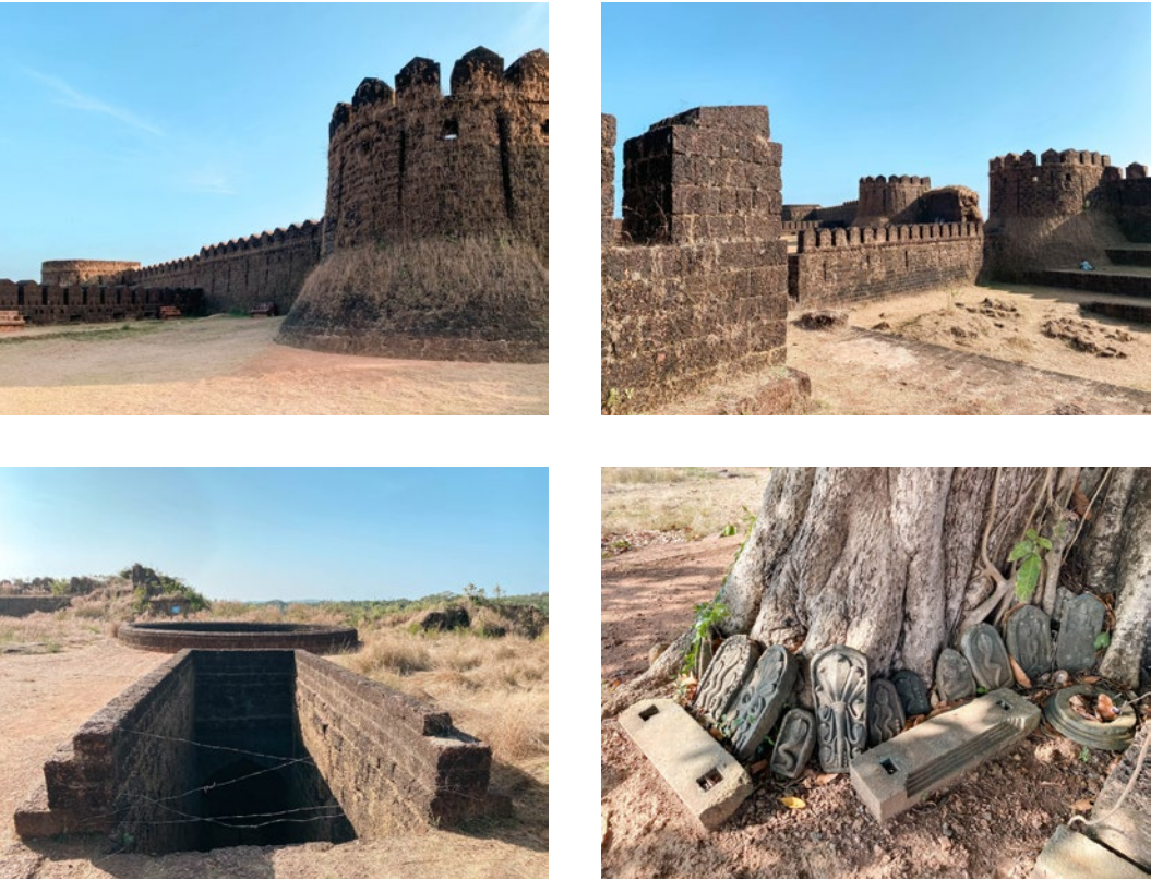
Glimpse of Mirjan Fort, built entirely from locally sourced laterite stones
