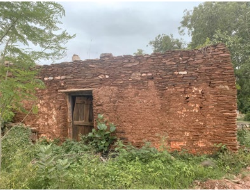
Clockwise from the top left: 1. Industrial Plant; 2. Presence of talcose argillite, a type of rock commonly found in the Hiriyur region; 3 & 4. An old dilapidated house with walls built using talcose argillite slate for masonry work
