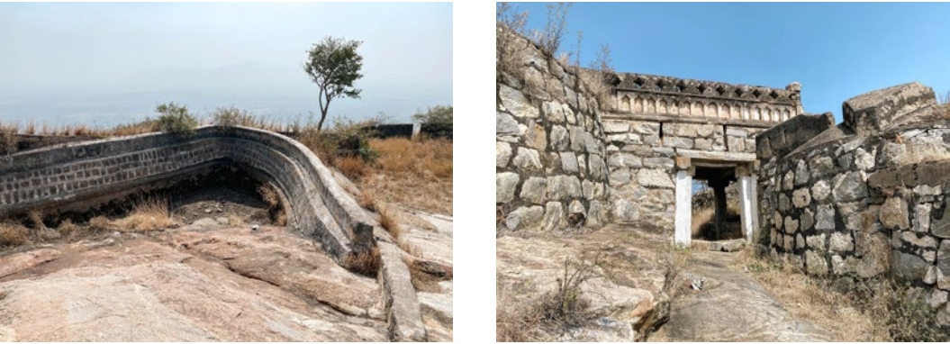
Clockwise from the top left: 1. View of Garudanagiri village from the top of the hill; 2. Defensive fort wall ramparts atop the hill; 3. The final fort wall gate at the summit; 4. A 'done' masonry structure built across the ridges to collect rainwater, serving as a water body for use in olden days
