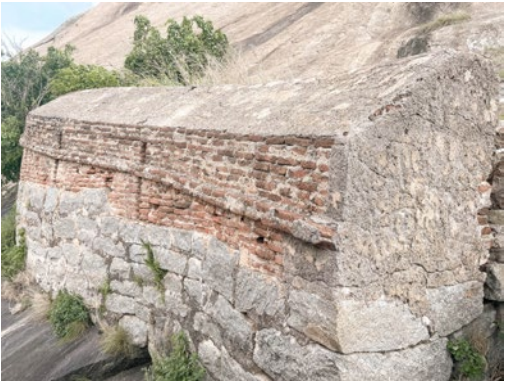
From the left: 1. A fort wall built on the granite slope of the hill; 2. A parapet wall constructed using granite stone, with brick and mortar detailing visible
