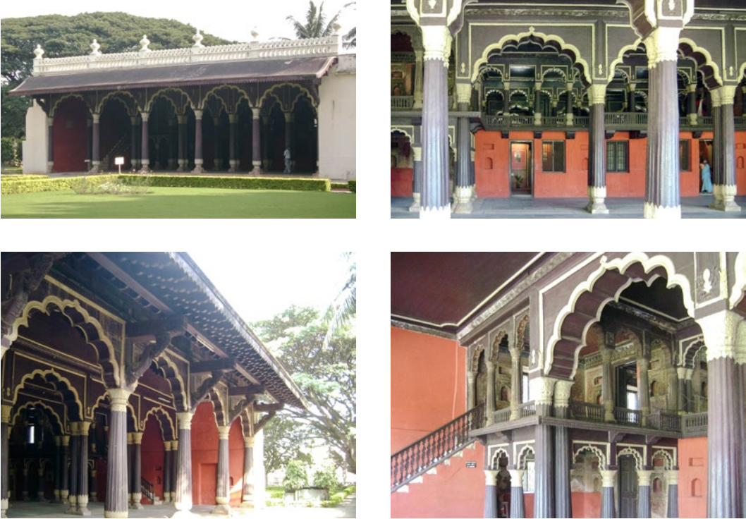
Tipu's Summer Palace is inside the Pete, near the Delhi Gate. The palace resembles the Daria Daulat, but unlike Daria Daulat, it doesn't feature many paintings inside. This palace was primarily built for his court (cutchery/office)
