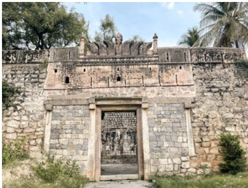
From the left: 1. A fort wall built on the granite slope of the hill; 2. A parapet wall constructed using granite stone, with brick and mortar detailing visible
