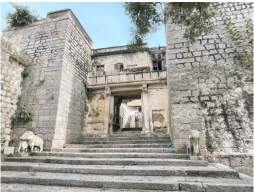
From the left: 1. A fort wall built on the granite slope of the hill; 2. A parapet wall constructed using granite stone, with brick and mortar detailing visible
