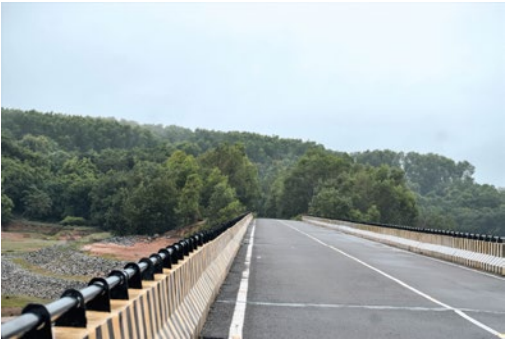
View of newly constructed Pataguppa Bridge
