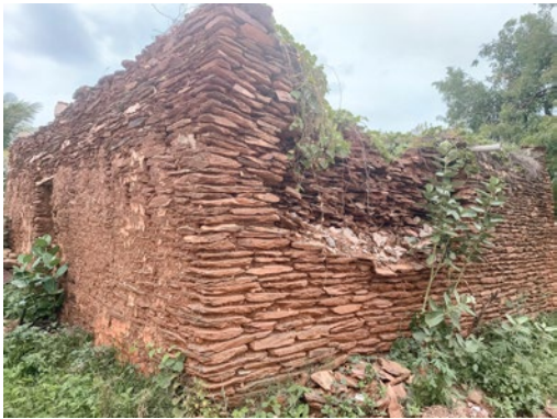
Clockwise from the top left: 1. Industrial Plant; 2. Presence of talcose argillite, a type of rock commonly found in the Hiriyur region; 3 & 4. An old dilapidated house with walls built using talcose argillite slate for masonry work
