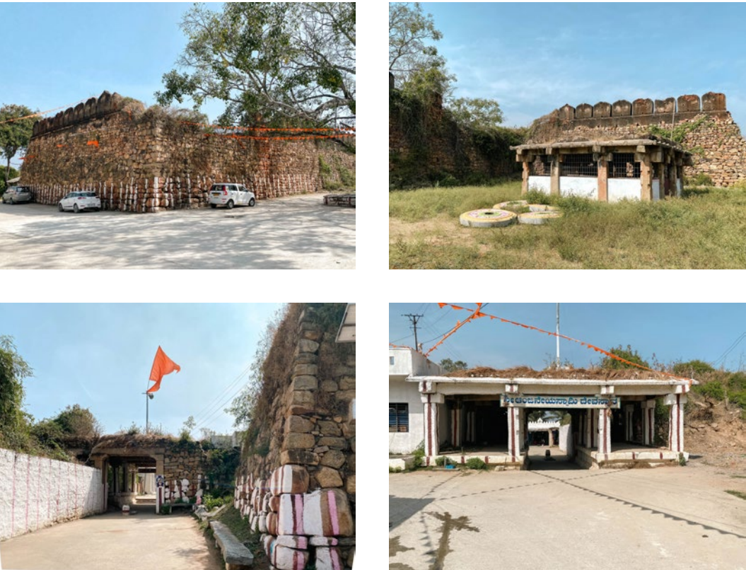
Clockwise from the top left: 1 & 2. The dilapidated fort structure, now in ruins and filled with debris and waste; 3 & 4. The Kote Anjaneya Temple near the fort entrance, along with the Kalikamba, Banashankari, and Channakeshava Temples, all of which remain accessible today
